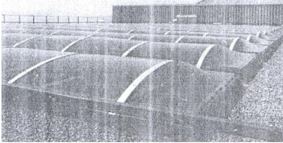
Figure 7.12: The suntrap of barrel sectioned “Plastilux” sheeting (Source: Crawford, 1978, page 37)
