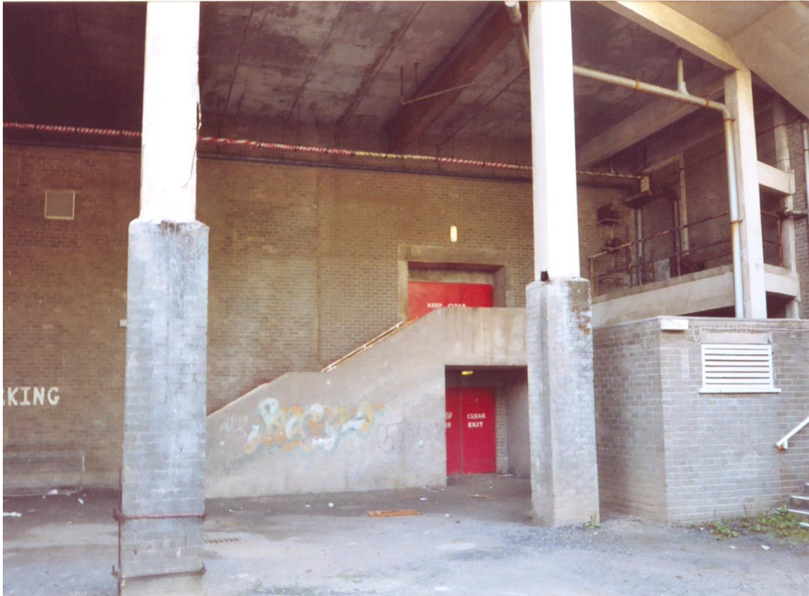
Figure 7.30: The point of discharge of the staircase (C1) serving the NE corner of the Piazza floor and the upper-level toilets is the lower of the two doors. This door can also be reached from the protected escape corridor to the north of the squash courts at Lower Downstairs Level (Photograph: Ian Phillips)
