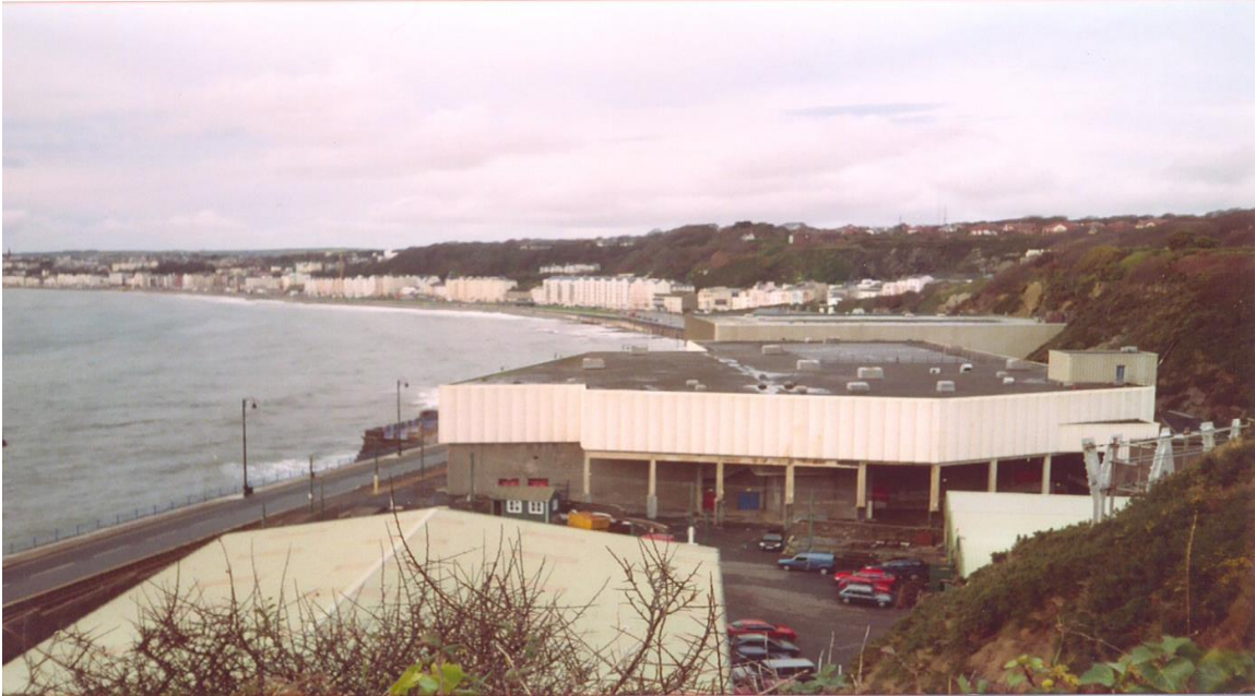
Figure 7.49: The authorities have gone to extremes in providing generous means of escape at Summerland's eastern end. Note that the roof height of the rebuilt Summerland is lower than the Aquadrome.
