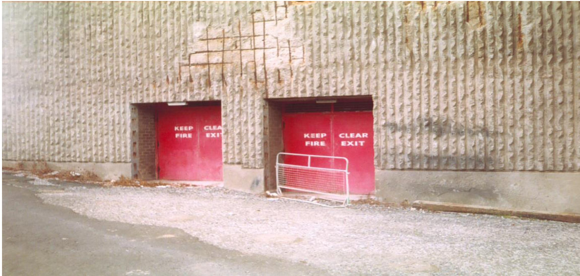
Figure 7.36: The SE enclosed staircase discharges directly into the eastern service yard (left-hand door). The fire exit on the right is from the sports halls. (Photograph: Ian Phillips)
