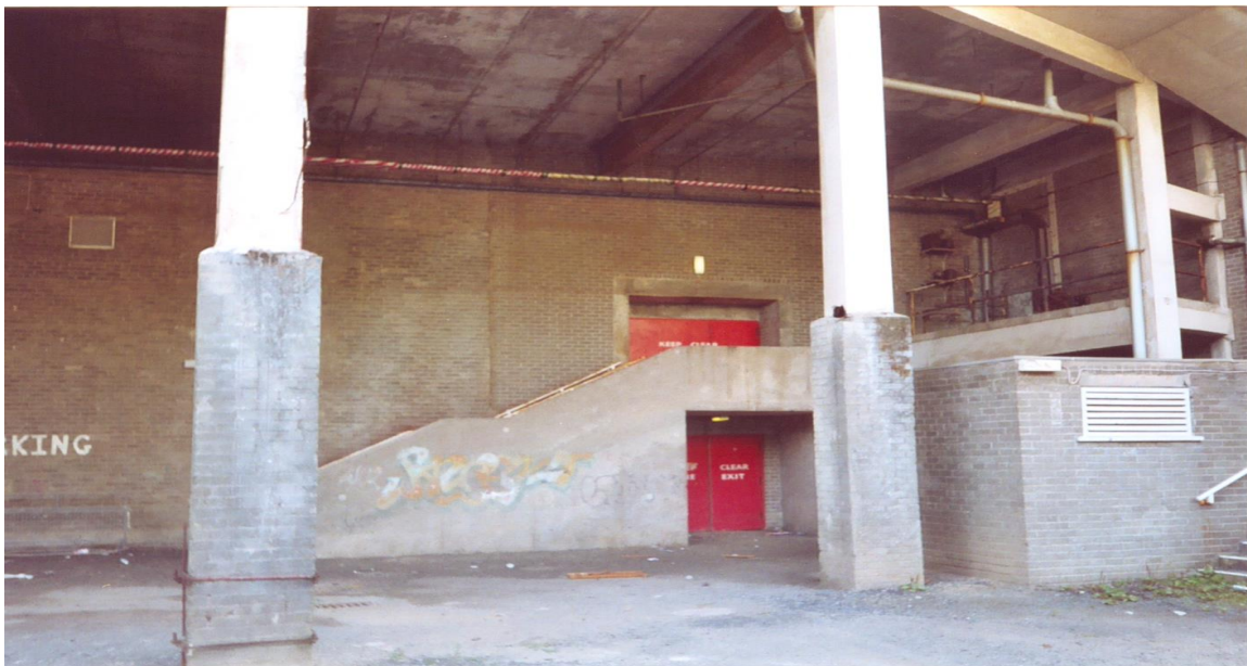
Figure 7.47: Two of the three fire exits (SQ1, SQ3) from the squash courts and their spectators' gallery. The third exit (SQ2) is out of view to the right of the ground floor fire exit visible in the photograph.
