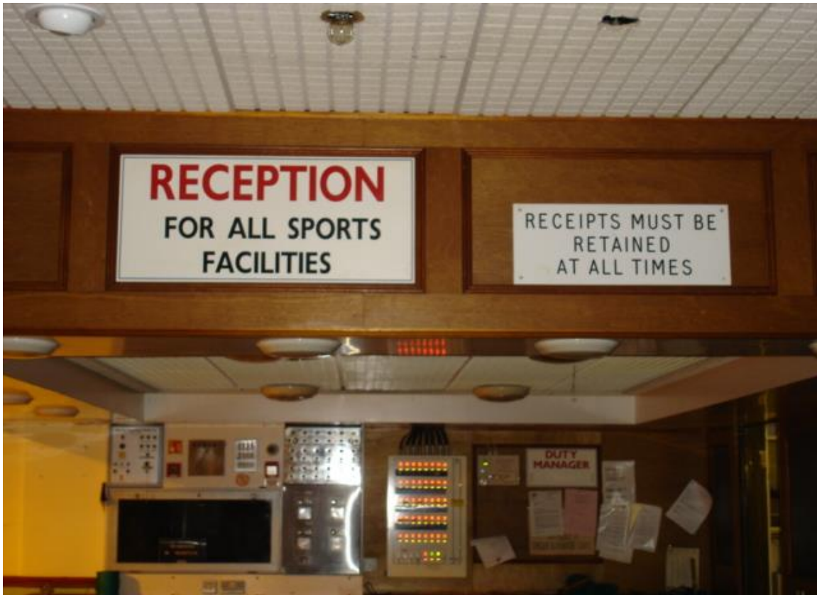
Figure 7.41: Reception desk containing Summerland’s central fire alarm panel. Note the ‘Duty Manager’ sign. (Photograph: Ricky Rooney and James Turpin)
