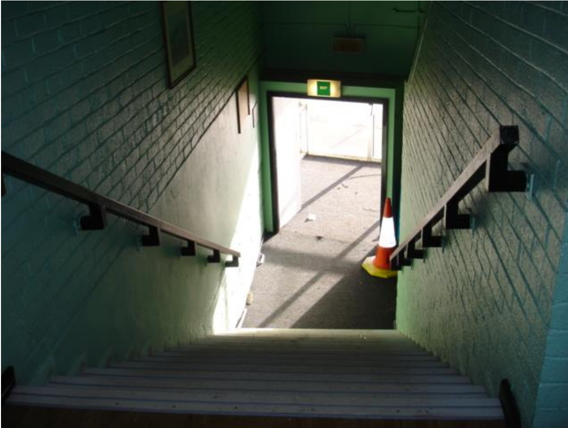
Figure 7.6: The staircase leading down to the main entrance. The doorway leading to the open air was only added after the fire. A person using this staircase in the original Summerland would have had to descend a further flight of stairs to the right of the traffic cone into the Disco Foyer area. This illustrates how escape routes in the original Summerland were not direct enough. (Photograph: Ricky Rooney and James Turpin)
