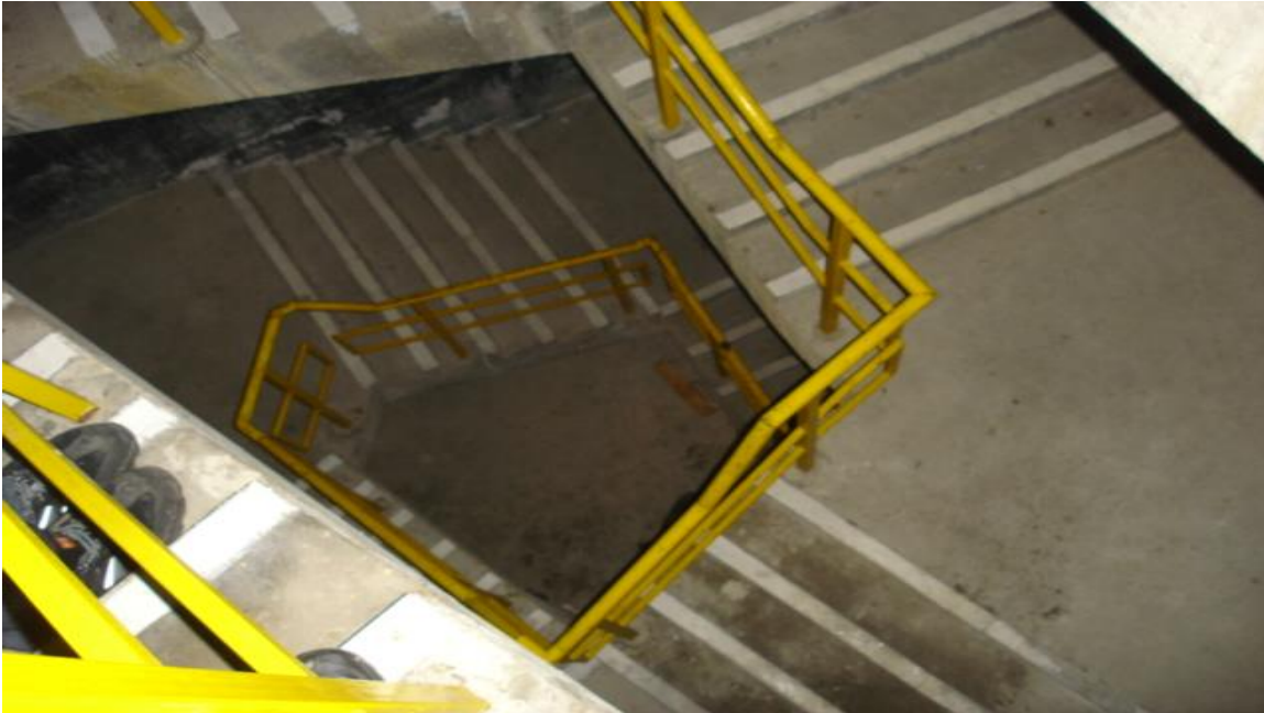
Figure 7.35: The SE Staircase. This staircase descends directly into the open air and can only be entered at Piazza floor level. Unlike the poorly designed NE Service Staircase in the original Summerland, the SE Staircase is a properly designed and sterile emergency escape staircase (Photograph: Ricky Rooney and James Turpin).
